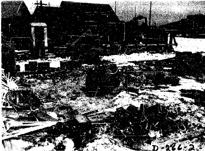
Fig. 3.9 Fire Damage to Tents (Origin I), 14-3/4 Miles from GZ
